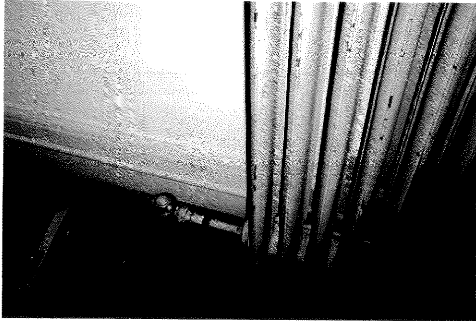
Cast Iron Radiator and Steam Trap
