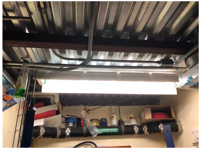
Ceiling of Janitor's Closet C117
