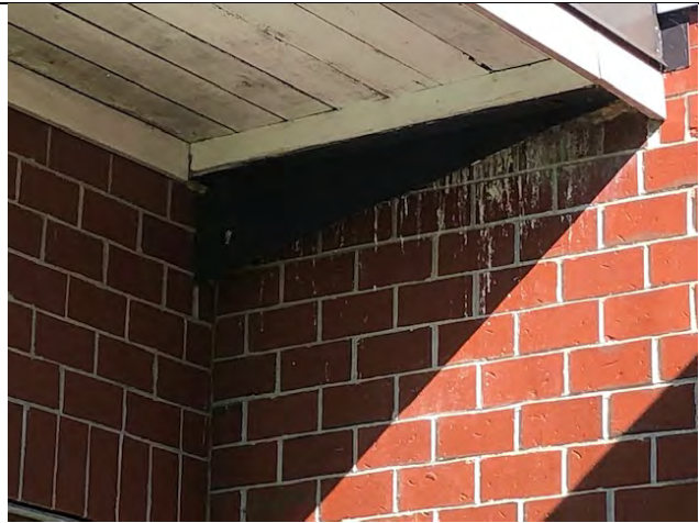
Figure A22: Exterior Wall Condition (EM)
