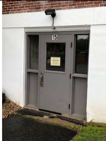
Figure A94: Door #15 (EM)
