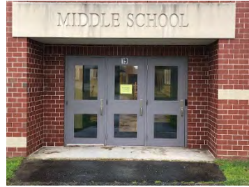
Figure A98: Door #19 (EM)
