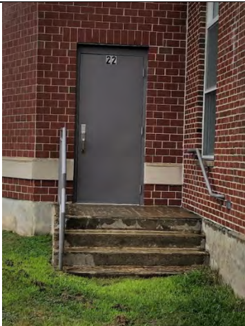
Figure A101: Door #22 (EM)
