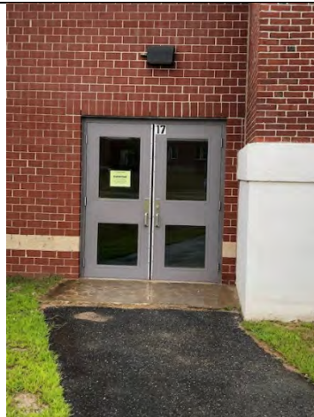
Figure A96: Door #17 (EM)
