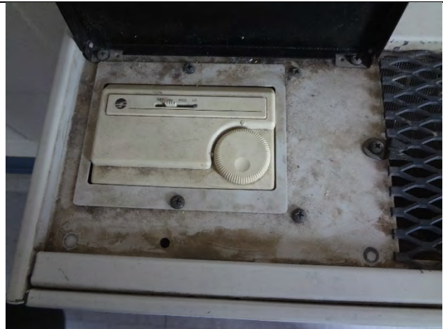
Figure H6: Clean & Repair Cabinet Unit Heaters (M)
