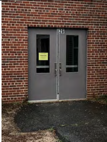
Figure A105: Door #26 (EM)
