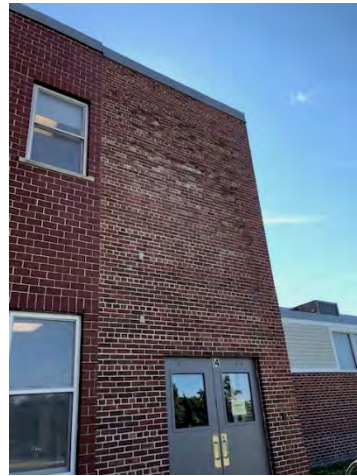
Figure A38: Masonry Repointing (EM)
