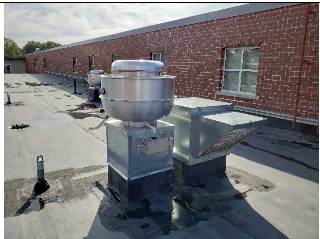
Figure H12: Screw Down Roof Equipment (EM)
