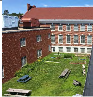
Figure A86: Courtyard without Compliant Egress, Conditions Issues (EM)
