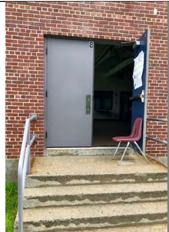
Figure A89: Door #8 (EM)
