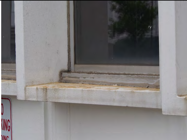
Figure A115: Precast Window System Sill (H)
