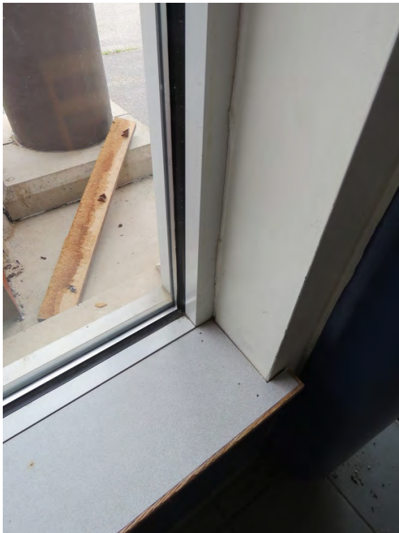
Window adjacent to entry doors at Pond Cove Entry D104
