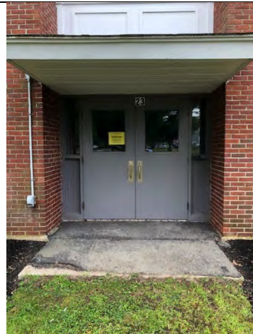
Figure A102: Door #23 (EM)
