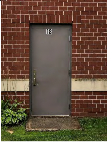
Figure A97: Door #18 (EM)
