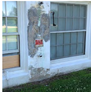
Figure A40: 1934 Building – Exterior Wall Condition (EM)
