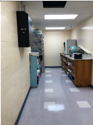
Figure A53: Non-ADA Protruding Object at Room E109 (EM)
