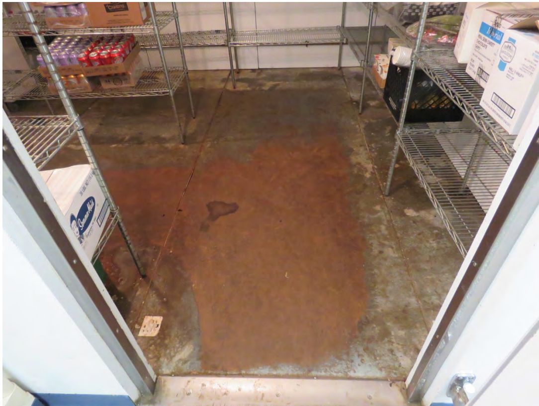
Kitchen cooler floor
