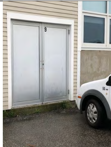
Figure A90: Door #9 (EM)
