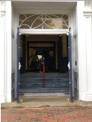
Figure A95: Door #16 (EM)
