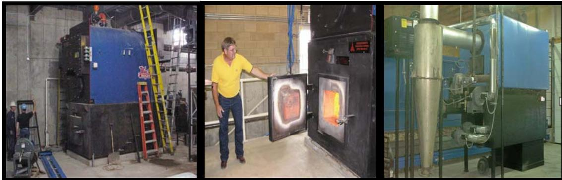
Figure 7 – Boiler, Combustor and Multi-Cyclone<sup>58</sup>
